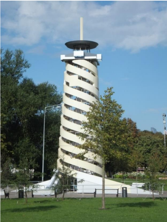
Figure 1: The Three Parachute Tower in Moscow's Gorky Park
